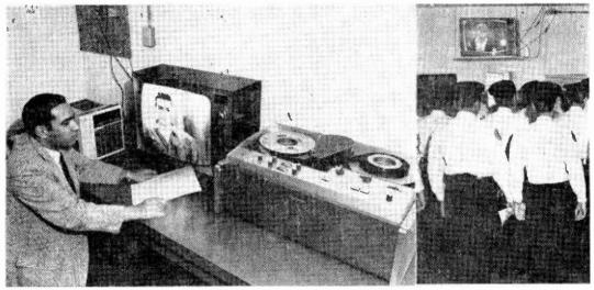
Ampex video tape system is used in experimental setup by Miami Police Department. Detective here is watching pre-recorded interview.
