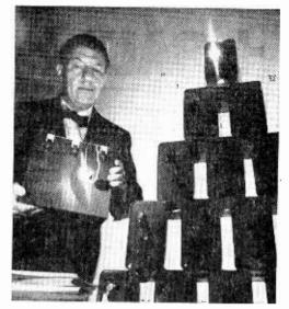
Single Magair battery packs as much power as stacked lantern batteries at right.
